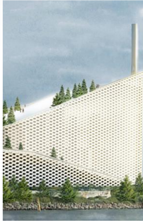
Waste incineration plants
