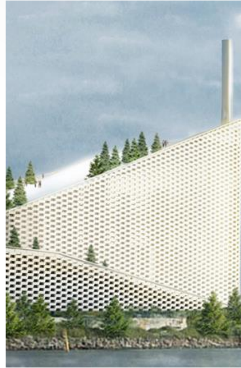
Waste incineration plants
